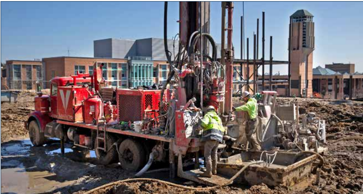
Figure 05. Geothermal drilling on Hayward Street
